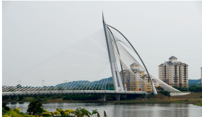
Figure 5. Seri Wawasan Bridge, Putrajaya, Malaysia, 2003.
