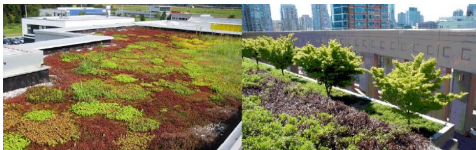
Picture 2: Extensive (left) and intensive (right) greening
