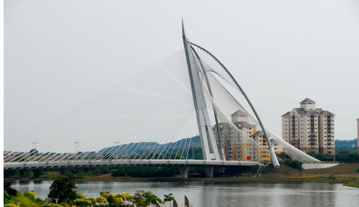
Figure 5. Seri Wawasan Bridge, Putrajaya, Malaysia, 2003.
